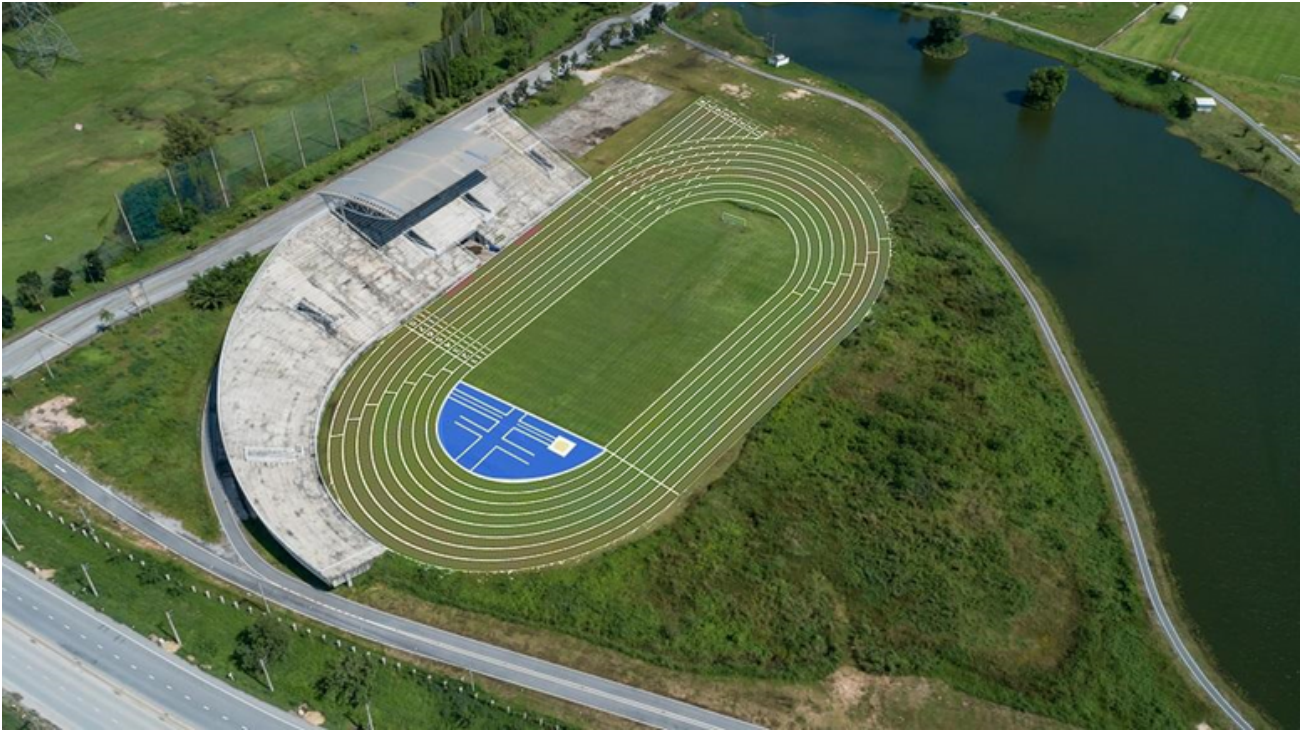
Top: 400m grass running track with rubberised area for high jump and long/triple jump with stadium seating.
